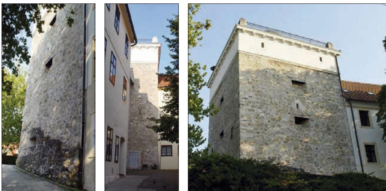
Fig. 47. Zagreb, Croatia – Pop's (Priest's) Tower (current state). View from the museum courtyard and from exterior, the tower has undergone extensions and modifications of window openings.
