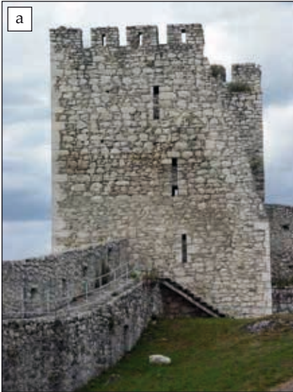
Fig. 53. a) Spiš Castle (Slovakia), tower (nr. 5), arrow loops with a shift for the defense of the fortification, lower gate and the access road to the castle, built simultaneously with the tower, covered with stone plates; b) Zadar (Croatia), Babja kula, a fragment of slit opening in the later modification of the interior; c) Hainburg (Austria), castle, entrance gate and Hainburg, town fortification.
