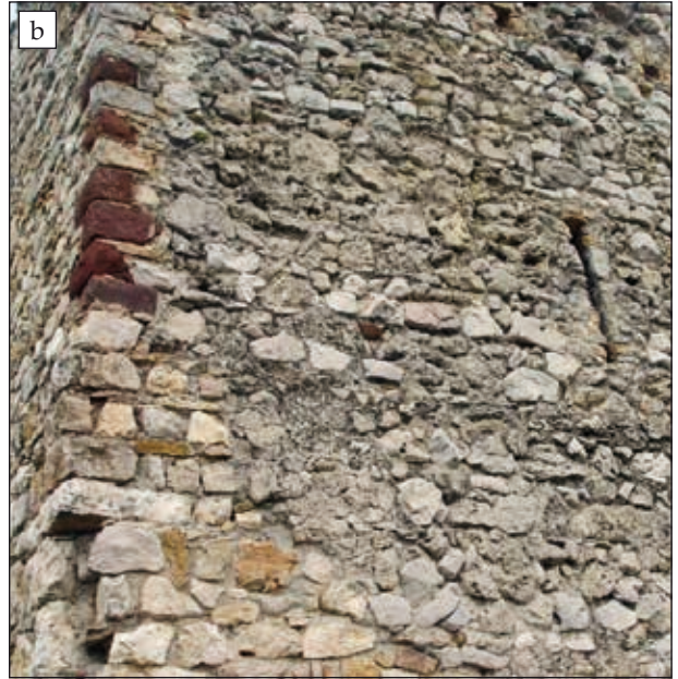
Fig. 52. The character of the tower walling – a) Blagoj (Croatia), b) Bánd-Esseg (Hungary), c) Korogvar (Croatia), Spiš Castle – Fioch's Tower (Slovakia), d) Spiš Castle – tower (nr. 5), e) Spiš Castle – northern wall of Provost's Tower.
