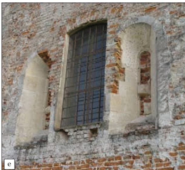
Fig. 40. a) Čazma – Southern façade with a pair of slit windows in a side nave and transept, b) Spišská Kapitula – slit window in the northern wall of the older, currently not extant transept above a later entrance hall, c) and e) Čazma – uncovered walled-in pair of slit windows of the transept, replaced by a later opening, d) Spišská Kapitula – Slit window in the northern wall of the transept – a detail, f) walled-in slit window in the southern nave under the top of the vaulting (under towers) at the time of the later annex of sacristy in the first half of the fourteenth century.
