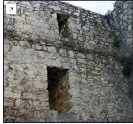
Fig. 53. a) Spiš Castle (Slovakia), tower (nr. 5), arrow loops with a shift for the defense of the fortification, lower gate and the access road to the castle, built simultaneously with the tower, covered with stone plates; b) Zadar (Croatia), Babja kula, a fragment of slit opening in the later modification of the interior; c) Hainburg (Austria), castle, entrance gate and Hainburg, town fortification.
