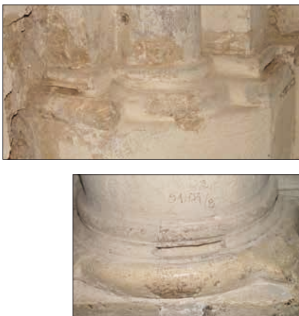
Fig. 29. Profiling of the base of a pier and a pillar, St. Martin's Cathedral, Spišská Kapitula.
